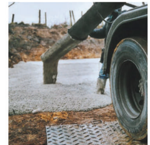
Ground-Guards provide the needed ground protection when concreting.
