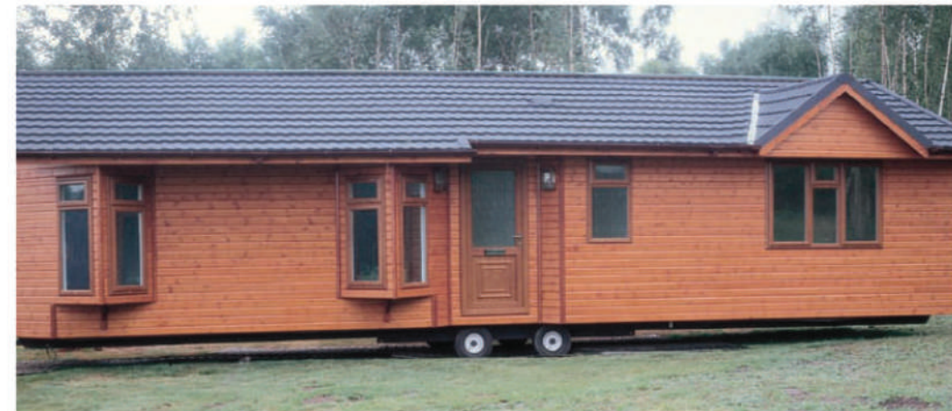
Siting this new 20 tonne two-part chalet home is made vastly safer and easier by the use of Ground-Guards.
