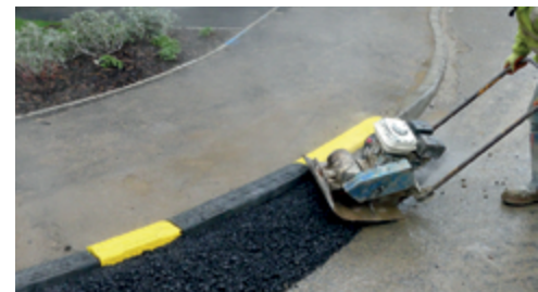
Haunch with temporary tarmac
